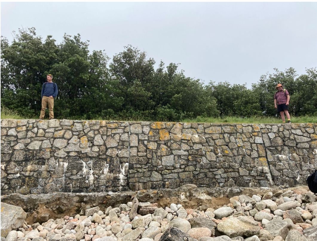
Figure 9.10: Scour erosion at the toe of the vertical wall
