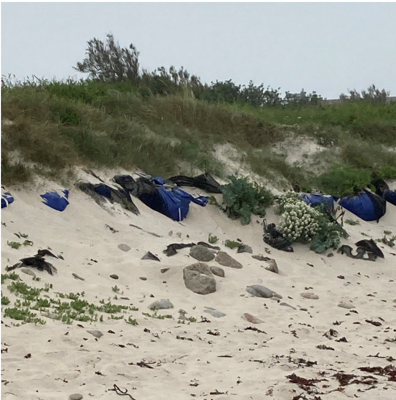
Figure 9.1: Exposed geobags at Periglis Beach
